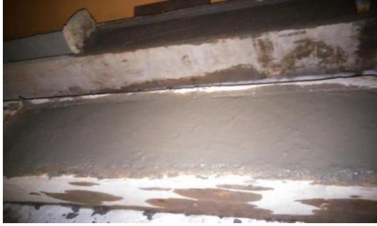
Figure 5: Casting of specimen
