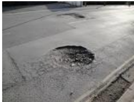
Fig 1. Condition of road with potholes
