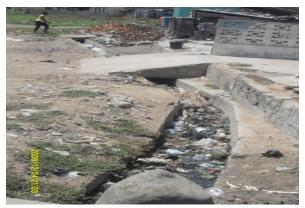
Plate 6: A choked gutter
